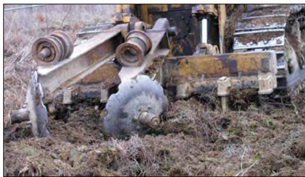
Figure 10-6.—Coulter wheels on the back of a dozer, with ripping tooth inserted into the soil. The coultter wheels pile loosened soil into a mound, allowing seedlings to be planted at a slightly elevated position above the land surface. Use of coultter wheels is advised for mine soils with poor water drainage and few large rocks. Photo by J. Burger, Virginia Tech, used with permission.
