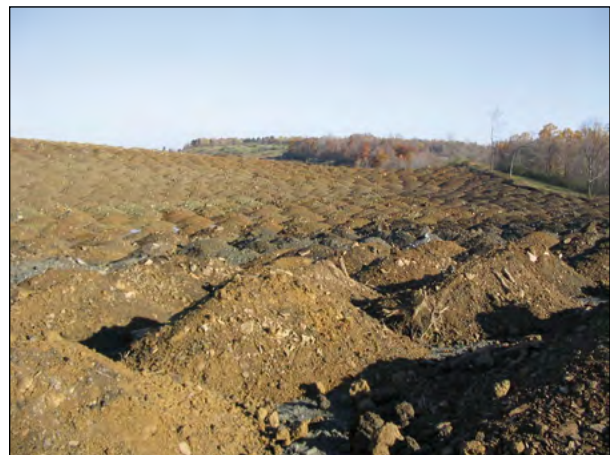
Figure 4-3.—Loose-dumped soils on the surface at an Ohio mine site. Photo by M. Hiscar, OSMRE.
