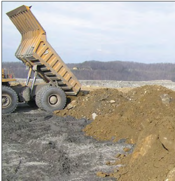
Figure 4-1.—Loose-dumping a topsoil substitute over a compacted subsurface on a West Virginia surface mine. The topsoil-substitute material is being dumped in closely spaced piles and will be graded using only a single dozer pass. The final surface will be revegetated with a tree-compatible ground cover and trees will be planted in the loose topsoil-substitute materials. Photo by J. Skousen, West Virginia University, used with permission.
