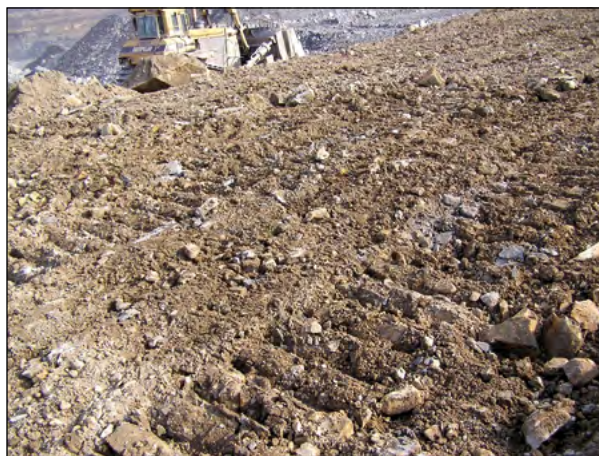
Figure 4-8.—A topsoil-substitute material that has been prepared for revegetation by using the low-compaction grading technique on a coal surface mine. The materials have been left in a loose condition. The rocky, rough surface will aid water infiltration and will not hinder the forest postmining land use that is being established on this site. Photo by J. Skousen, West Virginia University, used with permission.
