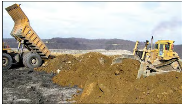
Figure 3-8.—Mixing of soil materials. Materials can be transported to the site, dumped in adjacent piles, and then lightly graded. Photo by J. Skousen, West Virginia University, used with permission.
